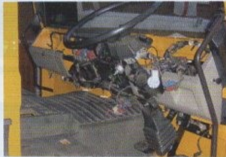
Fitting the interior to the new cab.
